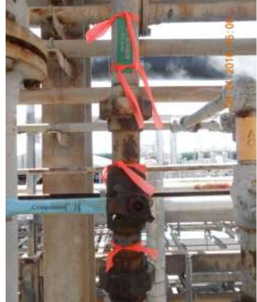
NPT Connection Leak Points
