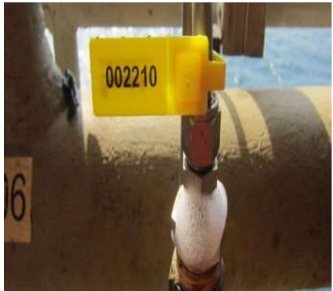
Threaded Connection Leak Points
