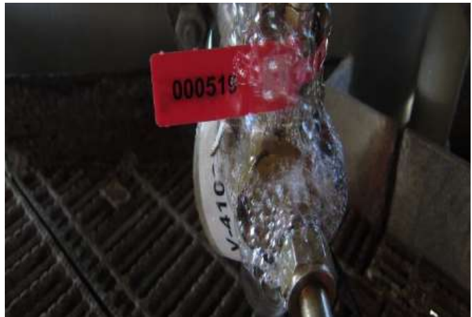
Leak Point with Tag
